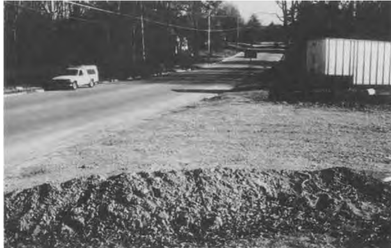
Figure 6.06a Gravel entrance/ exit keeps mud off public roads.
