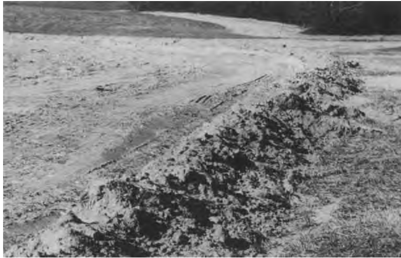
Figure 6.20a Temporary earthen diversion.
