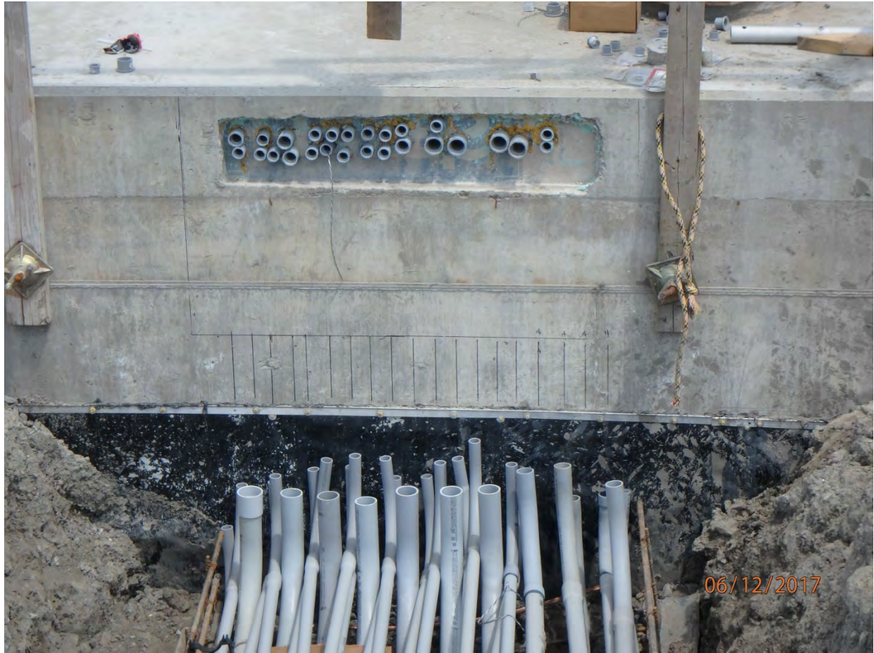
Photo 5 – Area behind and underneath wireway
