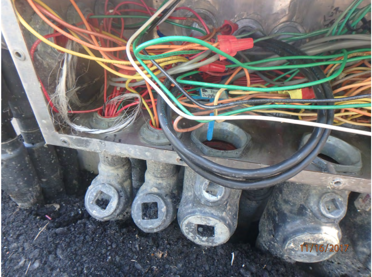
Photo 2 – Interior of wireway
