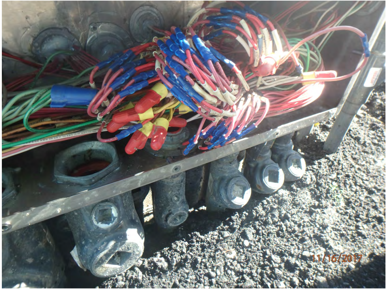
Photo 4 – Interior of wireway
