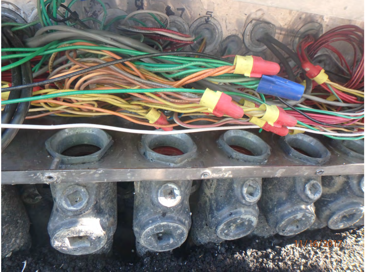
Photo 3 – interior of wireway
