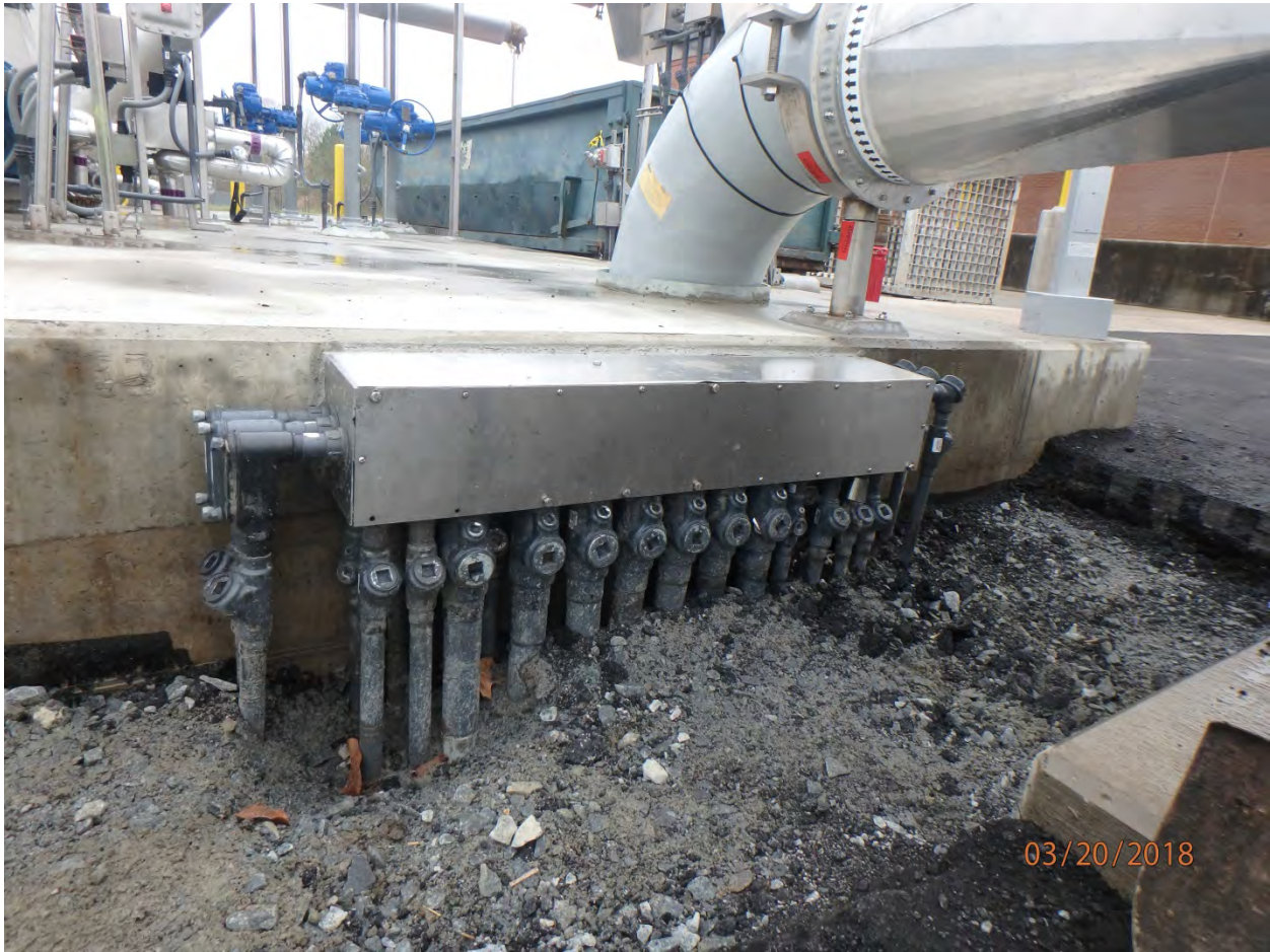
Photo 1 - Wireway to be replaced attached to southwest corner of screenings structure.
