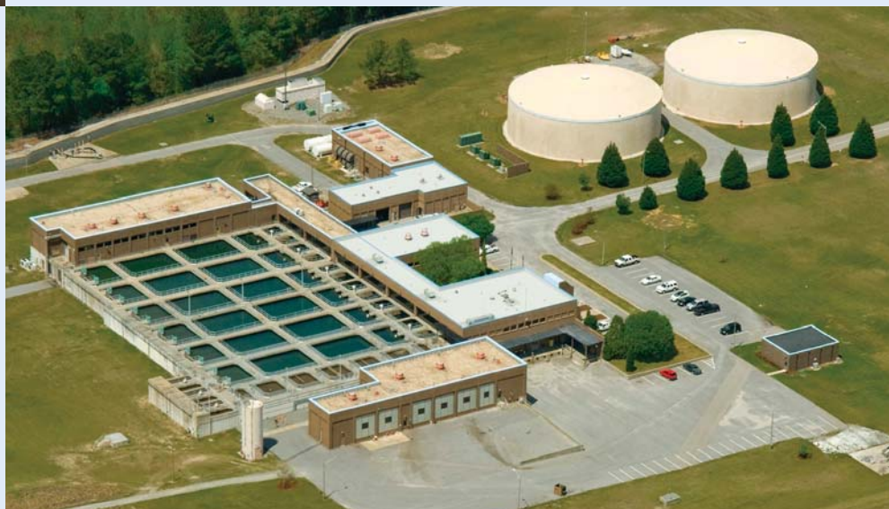
The Water Treatment Plant
