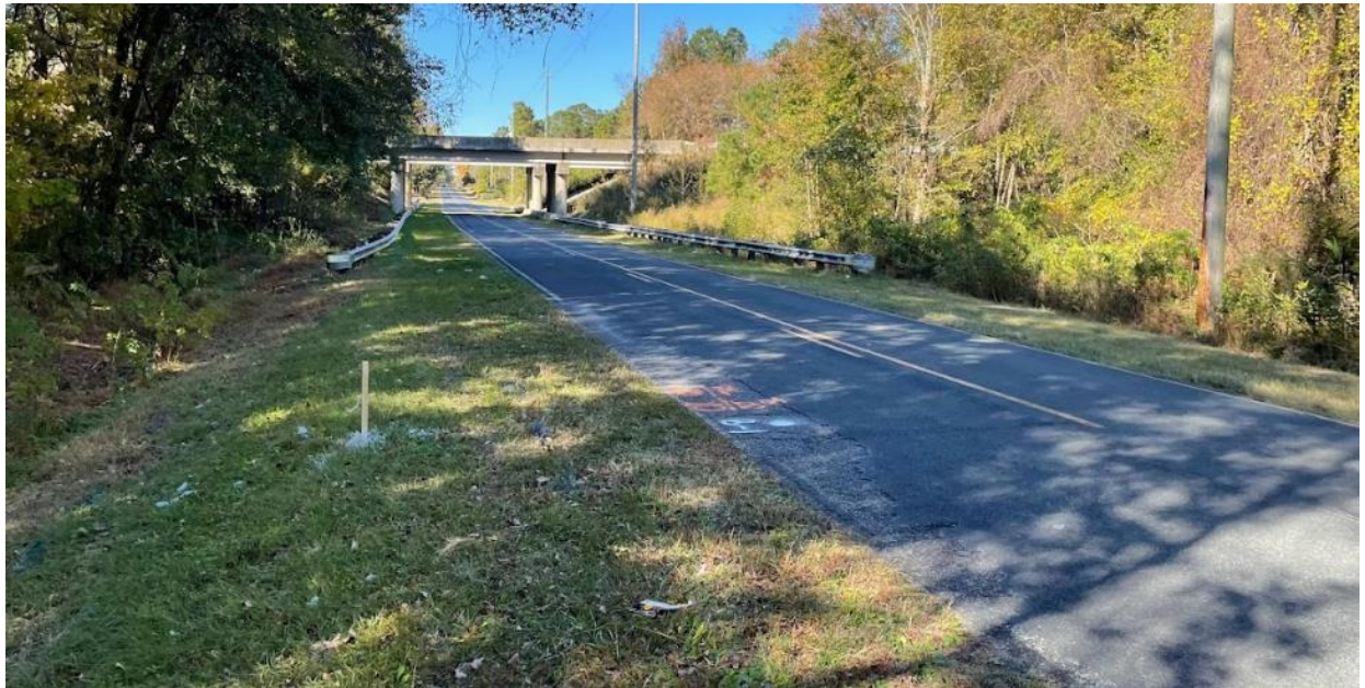
Boring B-1 facing north (B-1 was slightly offset southwest (further into the ditch) to avoid existing utilities, since this photo was taken)
