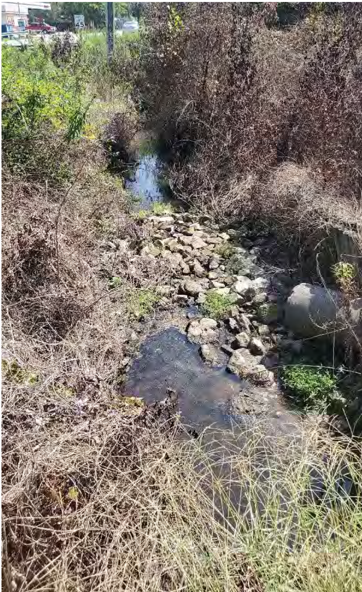
Photo 1. On southwest side of WLAA 1, facing east. Standing water is present in channel that discharges to adjacent creek.
